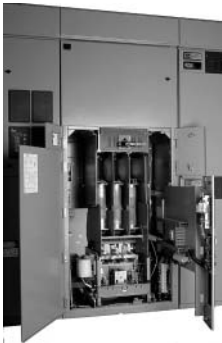
50L7 Vacuum Retrofit
